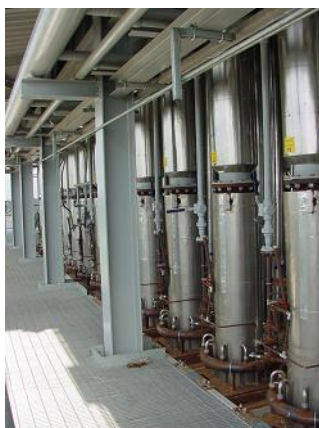
Figure 2. LSV™ burner installation.
